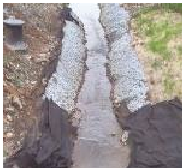
Figure 3.45. Construction of lined section of Mitchell Branch, MIK 0.7, in 1998
