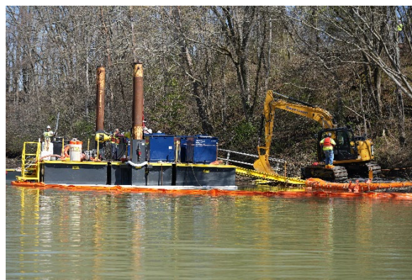
Figure 3.52. Workers excavate soil from the EU-19 mudflat to load on the floating platform
