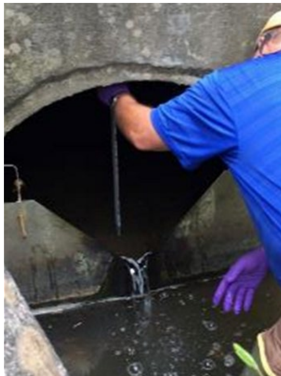
Figure 3.14. Storm water outfall monitoring
