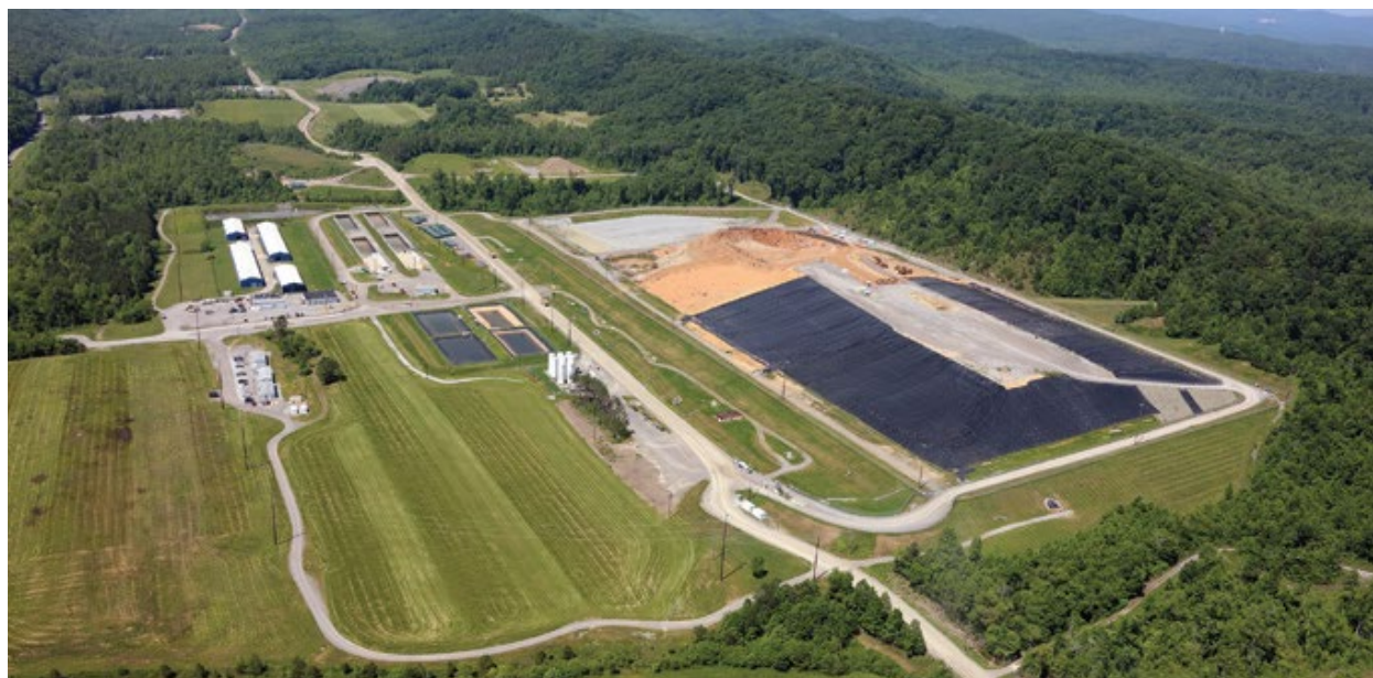
Figure 1.10. Aerial view of the Environmental Management Waste Management Facility
